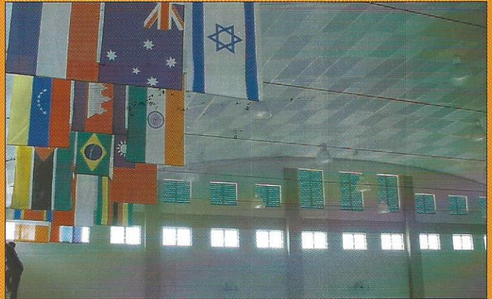
Interior Ceiling & Lighting
